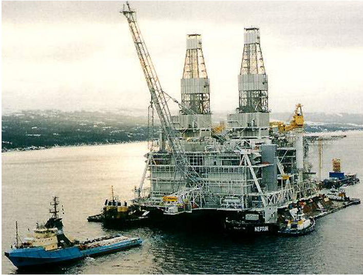
Figure 3: The Hibernia GBS being towed from its construction site at Bull Arm, Nfld.
