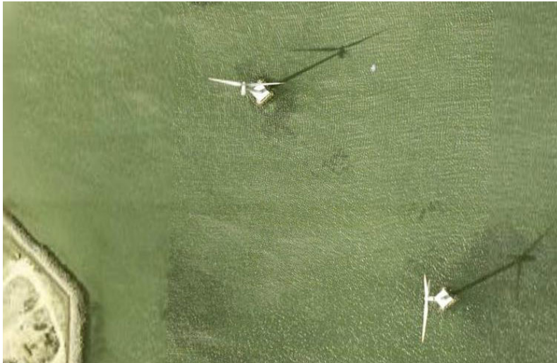
Figure 19: Offshore Wind Turbines – Denmark
